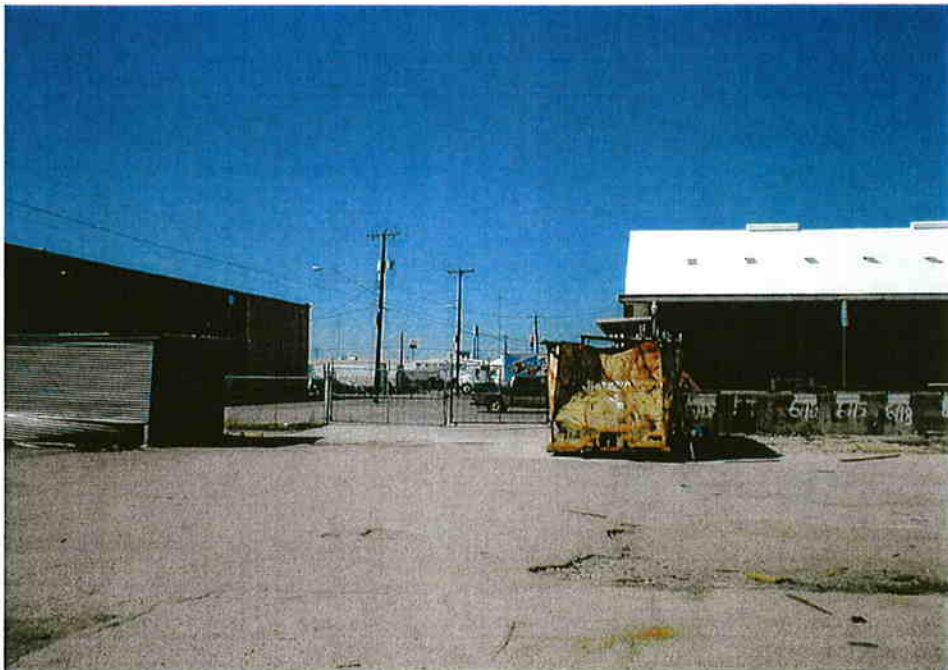
Photo #4: This photo shows a view of the storage shed, dumpster and loading dock area from the eastern paved parking/storage area.
