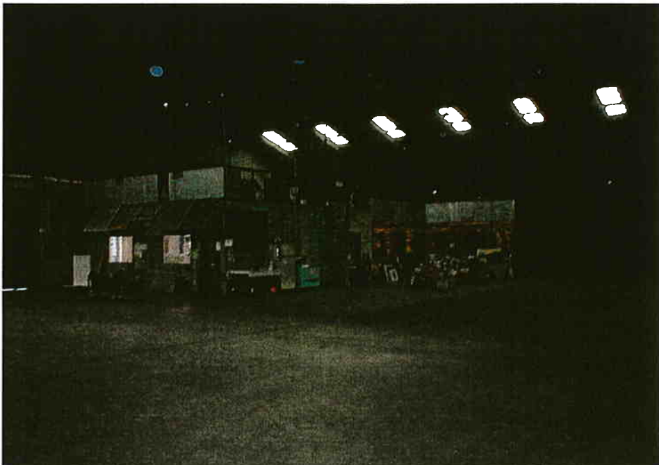
Photo #16: This photo shows a view of the interior of the warehouse building from the east, looking southwest.
