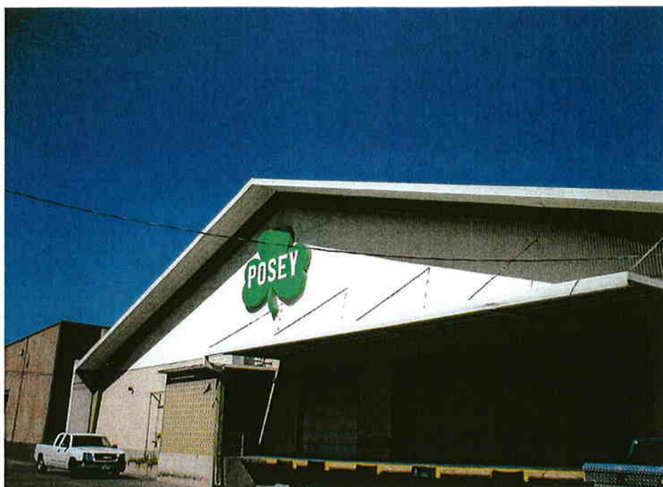
Photo #1: This photo shows the view of the front of the on-site metal warehouse facility from the southeast.
