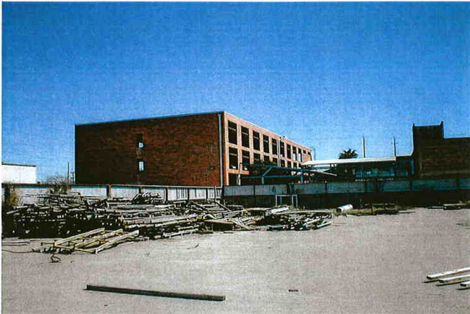
Photo #8: This photo shows the view of the northeastern portion of the site as seen from the loading dock area.
