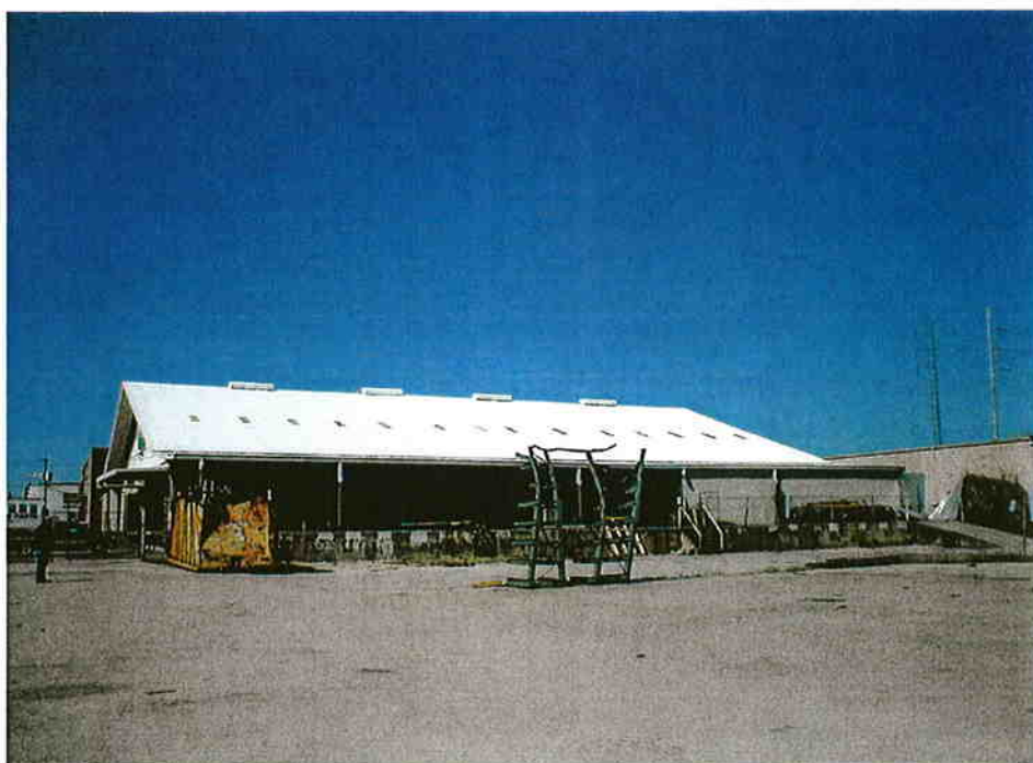
Photo #2: This photo shows the view across the site from the southeast.
