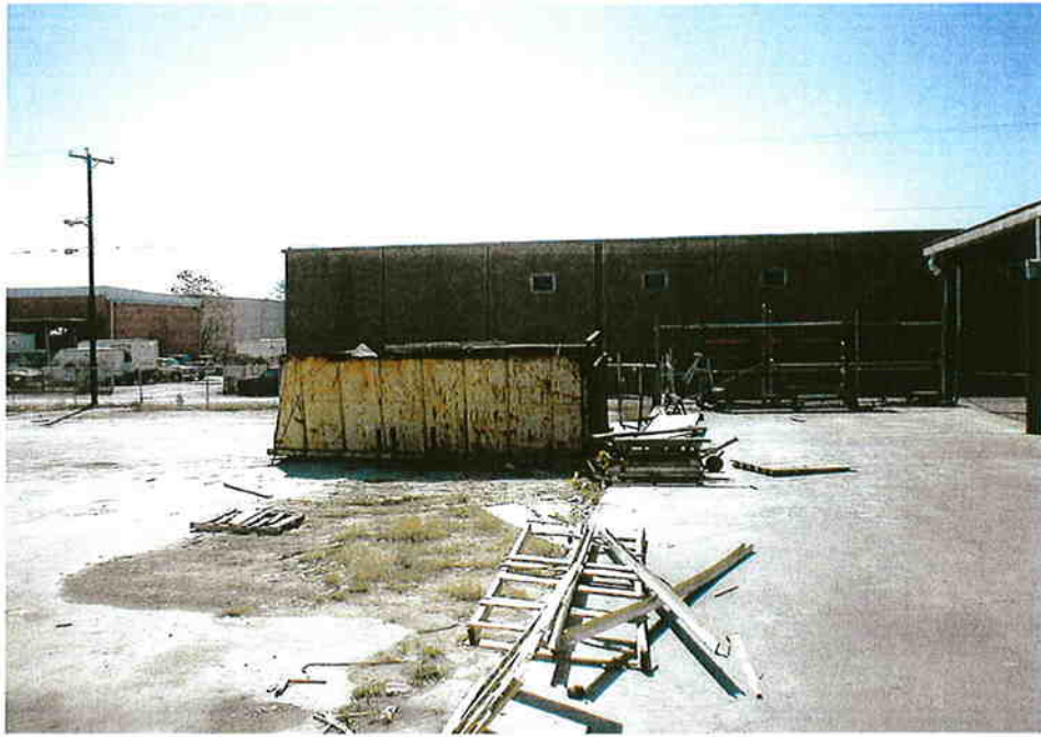
Photo #13: This photo shows the view along the loading dock area from the north.
