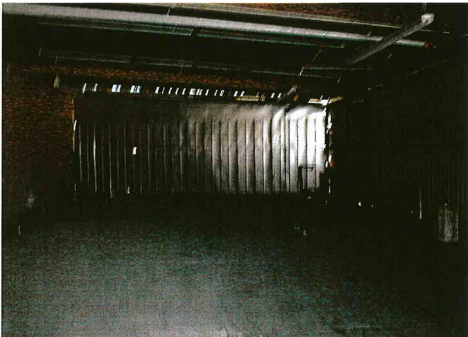
Photo #12: This photo shows the view along the covered portion of the loading dock area from the south.
