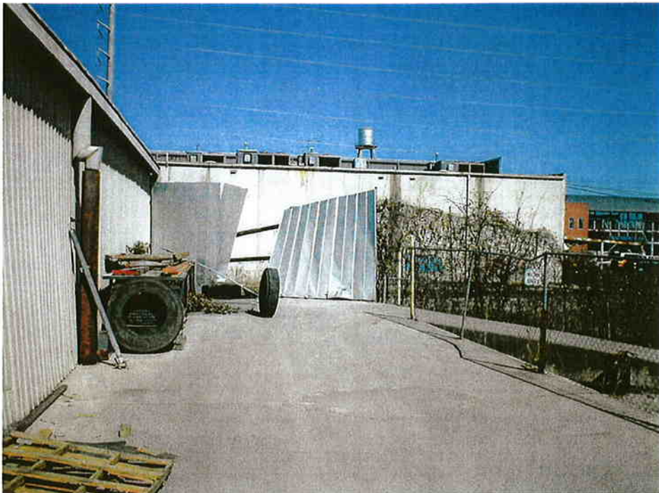
Photo #10: This photo shows the view north along the loading dock area.
