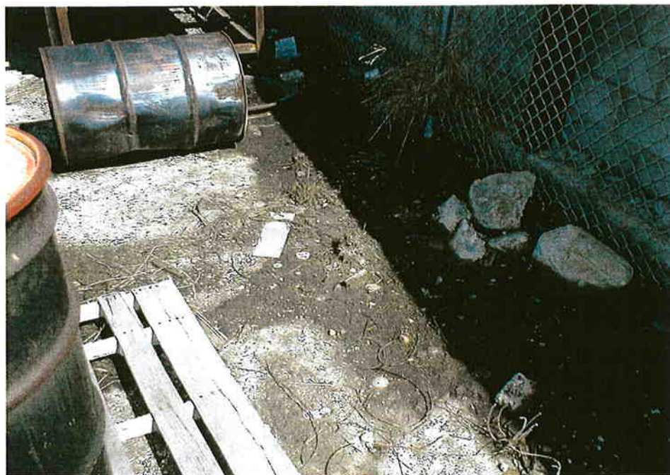
Photo #20: This photo shows another view of the surficial staining along the eastern boundary of the site.
