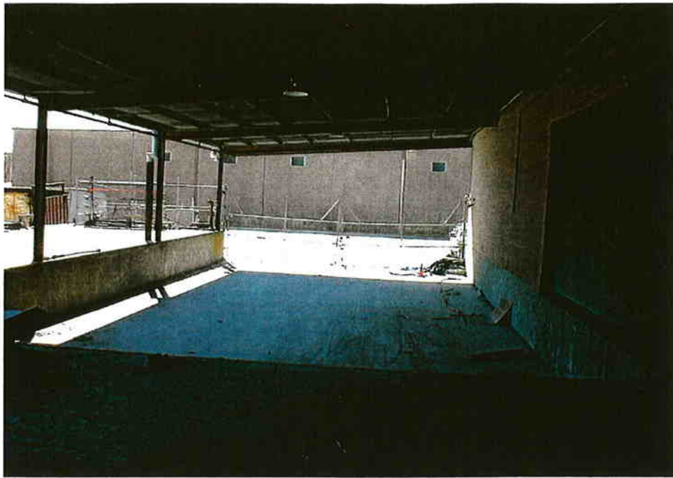
Photo #11: This photo shows the view along the covered portion of the loading dock area from the north.
