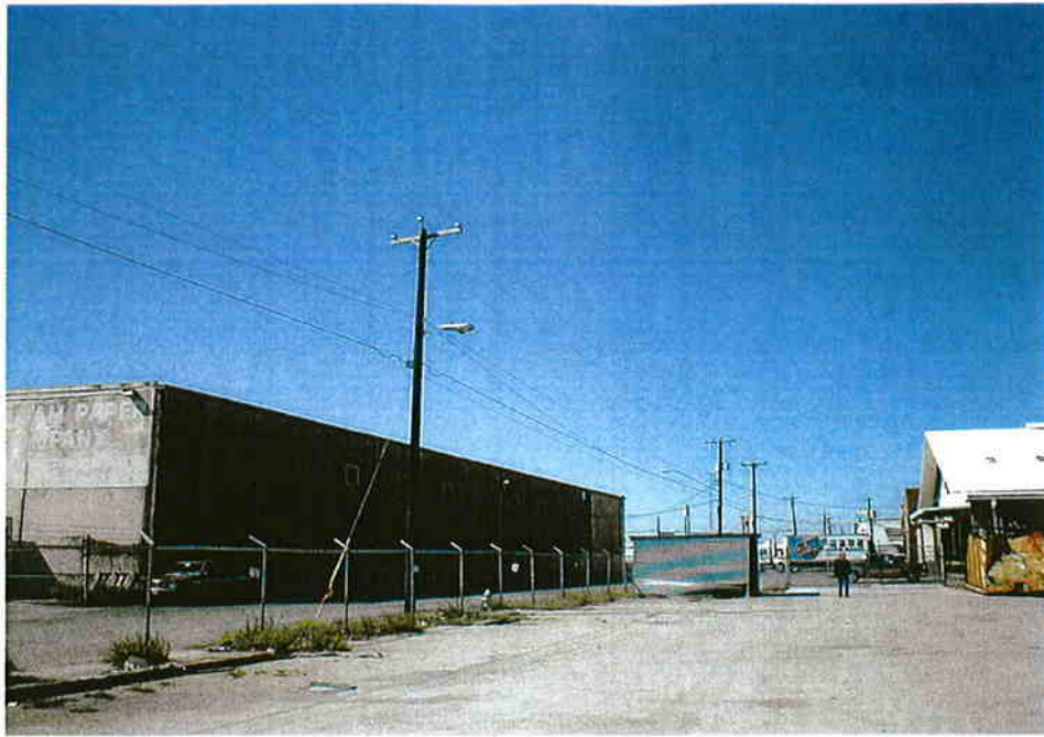
Photo #3: This photo shows the view across the site from the east, showing West Peden Alley and the adjacent warehouse facility.
